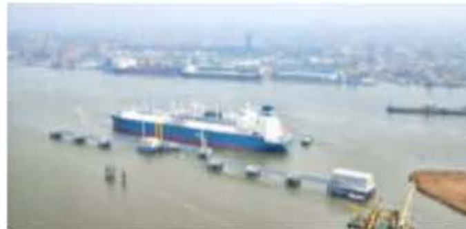
Klaipeda LNG terminal based on FSRU Independence
