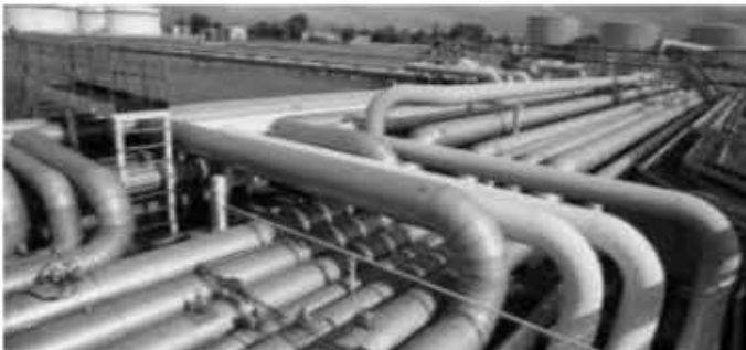
State fuel reserves terminal
