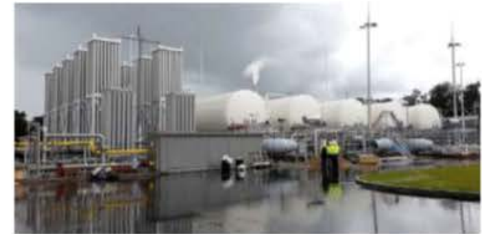
LNG reloading and bunkering station under construction in Klaipeda
